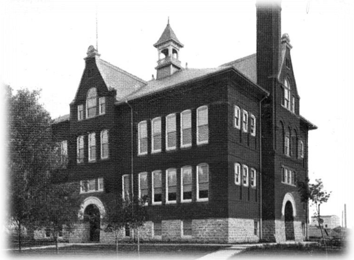
The new high school and grade school was completed in 1904 at a cost of $25,000. A renovation and addition was completed in 1936.
